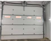
NUCOR All Steel Construction 21 x 45. Maintenance free standing seam 24-gauge roofing. Maintenance free inside all steel wall construction. 100 amp Electric service. 60,000 BTU high efficiency heater with thermostat. Six inches of insulation withR19 value in walls and ceiling. Two inch Clopay insulated R18, large 14 by 14 ft overhead door with windows [...]
