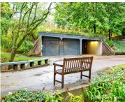
The "Underhill: Custom designed, energy-efficient, and sustainable house/design studio built in 1978. It is a passive solar, earth-sheltered, green-roof building explicitly configured to the topography of the hillside site. It features a zero-step main floor, is all-electric, and utilizes 100% renewable power from Consumers Energy (through the Green Generation program, Solar Gardens, etc.). There is [...]
