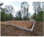
Barndominium under construction, expecting to finish mid September. This will be a one of a kind. Entire building with in floor heat on a full 4 ft. frost wall and insulated below the heat runs with 2 inch foam. Upper walls all 6 inch construction. All one level! Two Bedrooms and 2 full Baths [...]
